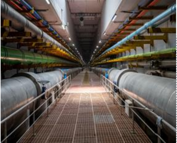
Underground Utility Tunnel
