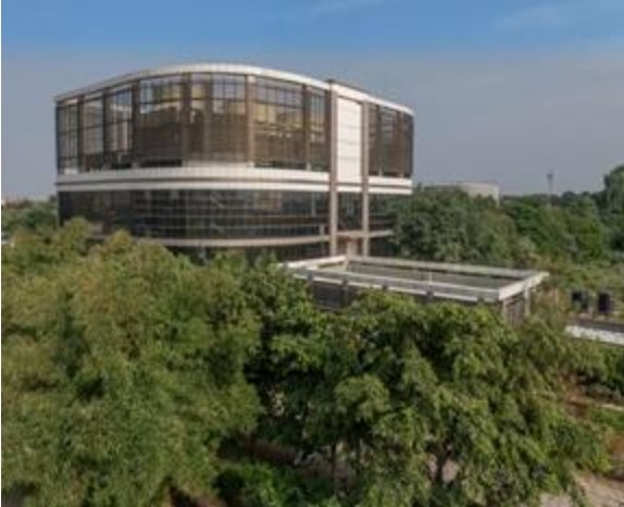
District Cooling Plant
