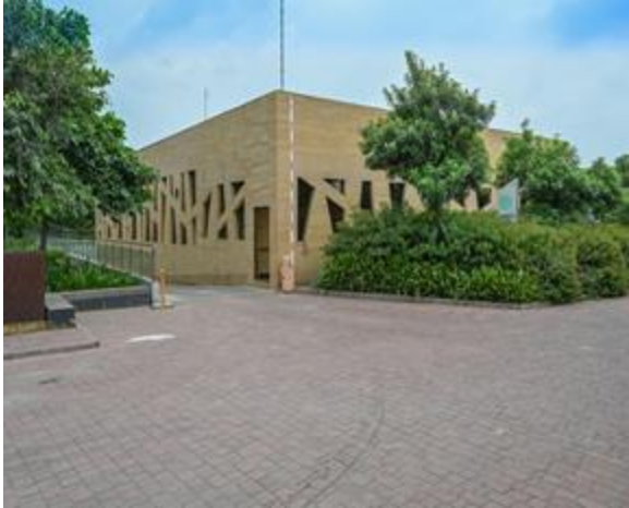
Automated Waste Collection & Segregation Plant
